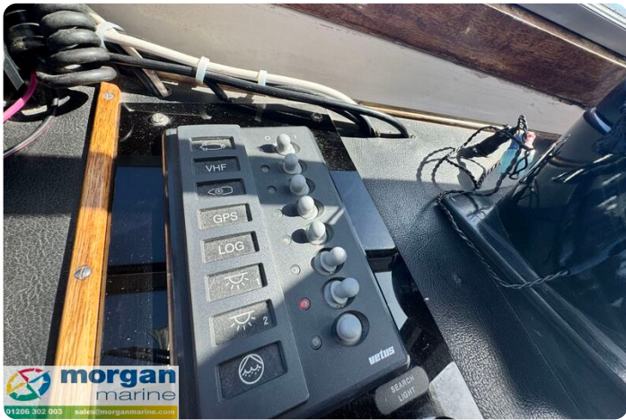
Aquastar 27 - switch panel
