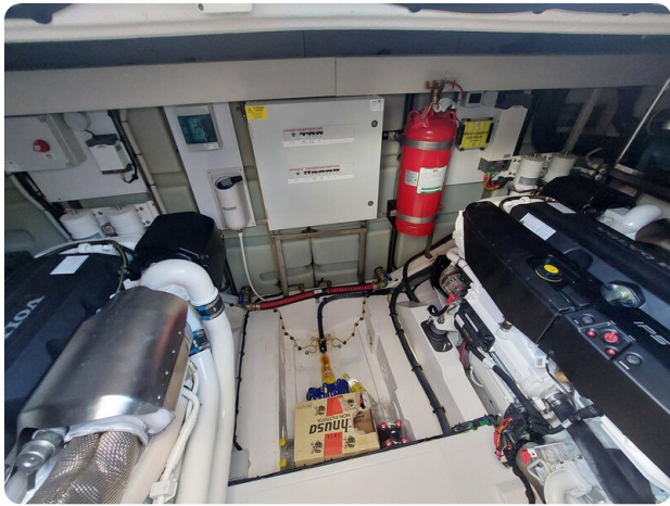
Azimut 53 Fly engine room
