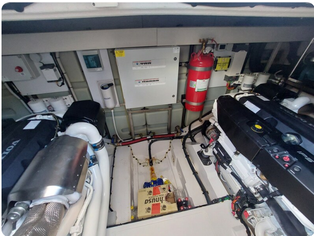
Azimut 53 Fly engine room
