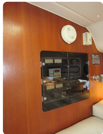
Tiara 3800 Open, electrical panel
